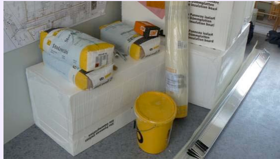
Insulation training : preparation of materials
